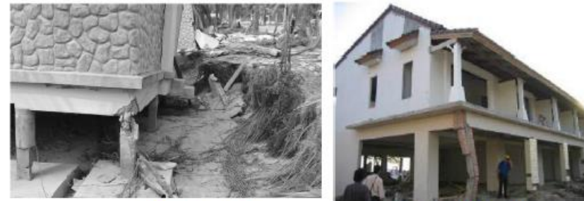
(a) Foundation failure
