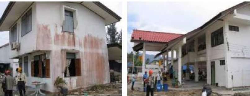
Figure 6.1 Damage Level 0 (No damage) for engineered RC building
